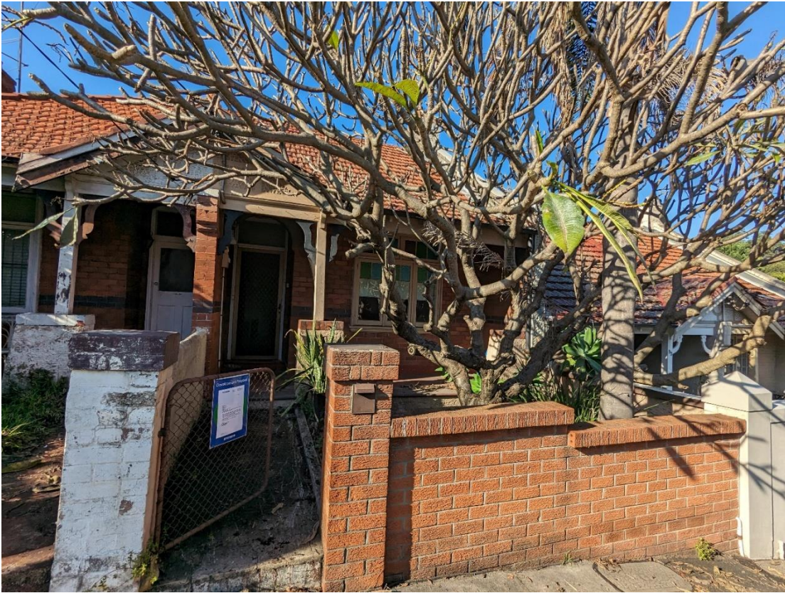
Figure 3: Site viewed from Wigram Road facing southeast
