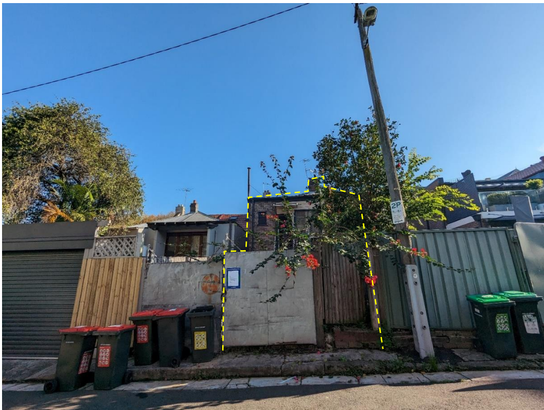
Figure 8: Site (outlined yellow) viewed from Wigram Lane
